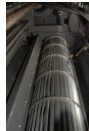
13-in. (330 mm) max flow fan in A85 provides high volume and low pressure air supply.
